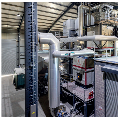
(Above) All material, boiler fuel for the CHP plant, and pellet feedstock, is trucked to the site. A JCB 560-80 Telehandler loading sawdust into the pellet plant receiving bunker. (Centre) Inside the spacious boiler house, the 4 MWth Kolbach boiler sits on raised frame. (Left) The split level pelleting line with the Stela belt dryer and CPM press on the upper level.
